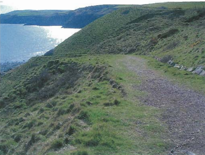
Most of the trackway is still in reasonable order
