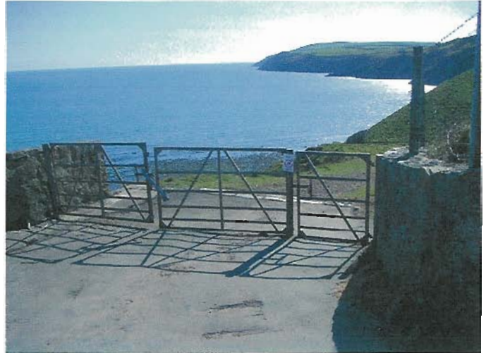
The access gate- locked since 2001
